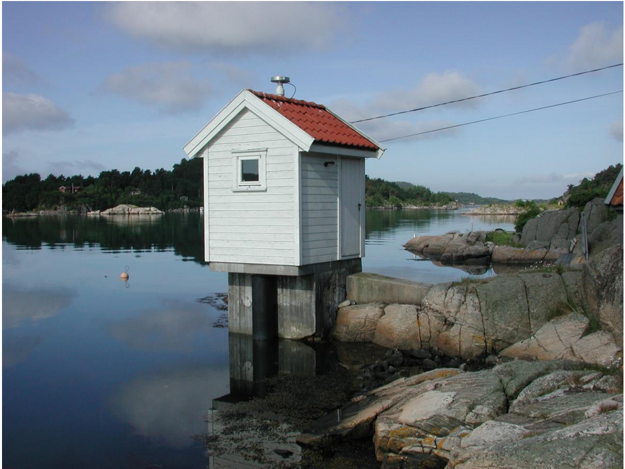
Figure 3. The house of the tide gauge at Tregde.
